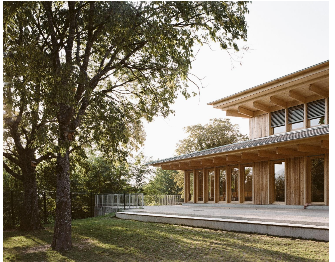
ECOLE A CHAMBERY BRENAS DOUCERAIN ARCHITECTES
